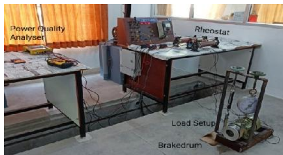
Fig. 3.1(b) Experimental setup for load testing of three phase induction motor
