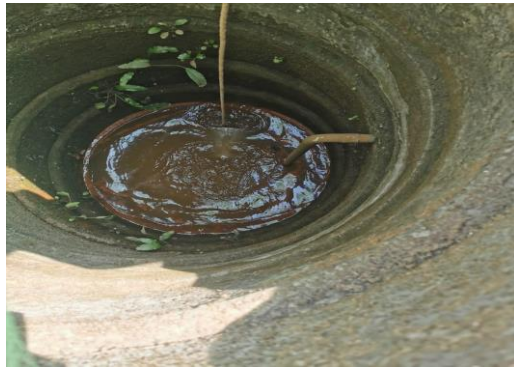
Fig 3. Unused well due to pollution
