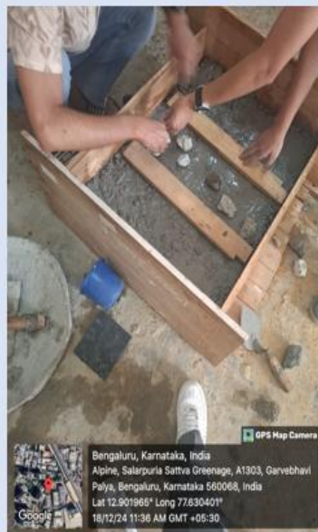
Placing concrete
